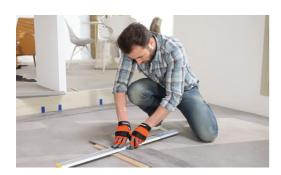
4. Then you can start the second row. The  $1^{st}$  plank of the second row should be smaller than the  $1^{st}$  plank of the  $1^{st}$  row to create a staggered installation. To do so use the rest of the cut last plank of the  $1^{st}$  row or use a new plank which you should cut so that it is smaller than the  $1^{st}$  plank, but no shorter than 30cm.
