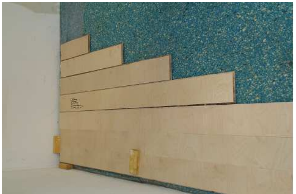
Cut the Lumaflex panels in order to obtain an homogeneous resistance Before assembling (the 3 first strips on this photograph)
