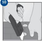
The board's short end meets a pipe: Drill a hole at least 16 mm larger than the diameter of the pipe. See Expansion gaps section. Then cut the board across through the hole.
