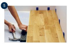
First join the long side, then the short end. Use Tarkett's tapping block when joining the boards together.
