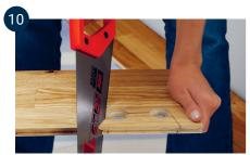
Saw off the piece to be placed behind the pipes, closest to the wall. Cut at an angle as shown in the image. If the pipe is located at the short side of the floor, the board must be cut at a 90° angle straight through the holes.
