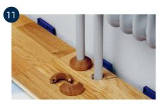
Knock the board into place, glue on the loose piece, place a wedge against the wall and cover with pipe collars.
