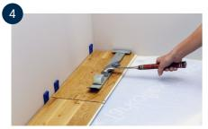
Then cut the board. Glue the short end, slide the board into place, hit them together with the Tarktool percussion iron, and fit a wedge at the short end against the wall.
