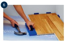
Use Tarkett's tapping block when joining the boards together. Tip: If the rows of boards are long, it is difficult to fit the board wedges after the first row. Therefore, wait until 4-5 rows have been laid, use Tarktool, and push the laid platform away from the wall before fitting the wedges.
