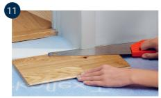
Door linings can be removed and moved up, but it is usually easier to saw them off. Use a loose floor board as a height template, and saw the lining with a fine toothed saw. Slide the floor under the liner. Make sure that the floor is not pinched between the substrate and the lining.
