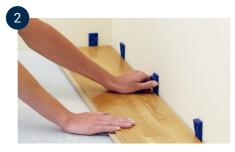
First row. Remember that the floor boards should preferably be laid in the longitudinal direction of the room. Start in a left corner with the tongue side against the wall and work to the right. Press down wedges between the floor and the wall to create an expansion joint of at least 8-10 mm.
