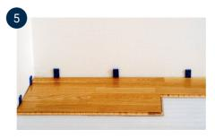
First board, second row. Start with the cutoff board from the first row. Note that there must be at least 500 mm between end joints over the entire floor (at least 300 mm for < 1.250 mm long boards). This does not apply to start & stop boards.
