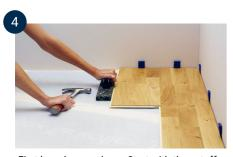
First board, second row. Start with the cutoff board from the first row. Note that there must be at least 500 mm between end joints over the entire floor (at least 300 mm for < 1.250 mm long boards). This does not apply to start & stop boards.
