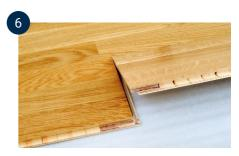
Second board, second row. Carefully place the board close to the short end of the previous board.
