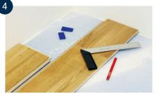
At the end of the row, turn the last board so that the groove side is against the groove side. Push the short end tight against the wall. Mark the cut with a pencil, at least 8-10 mm from the short end of the previous board, so that you have an expansion joint when the board is put in place.
