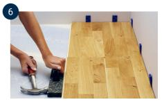
Tip: If the rows of boards are long, it is difficult to fit the wedges after the first row. Therefore, wait until 4-5 rows have been laid, use Tarktool, and push the laid platform away from the wall before fitting the wedges.
