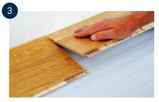
Second board, first row. Carefully place this board close to the short end of the first board. Then press or tap lightly on the short end that has just been laid.
