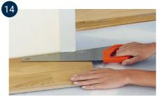
Door liners can be removed and moved up, but it is usually easier to saw them off. Use a loose floor board as a height template and saw off the lining. Make sure that the floor is not clamped between the subflooring and the frame.
