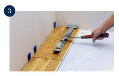
Then cut the board, slide the board into place, hit them together using the Tarktool percussion iron, and fit a wedge at the short end against the wall.
