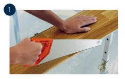
Before laying the first row, you must cut off the protrusion on the tongue side.
