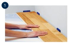
Lay out the first row of boards. Start with the groove side against the wall and work to the right. It is very important that the first row of boards is straight.
