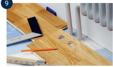
If the long side of the board meets a pipe, drill a hole with a diameter of at least 16 mm larger than the pipe's diameter, so that there is an expansion joint around the pipe. Use a pencil to mark where you want to saw.
