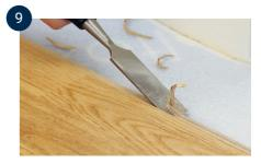
If there is not enough space to fold down the last board (e.g. door liner, radiator), it can be pushed in from the side instead. To make this possible, the protruding lip of the previous row of boards must be straightened. Use a chisel to cut off the part of the lip that is protruding at the top of the outer edge.
