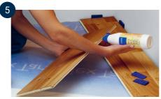
First board, second row. Start with the cutoff board from the first row. Note that there must be at least 500 mm between end joints over the entire floor (at least 300 mm for < 1.250 mm long boards). This does not apply to start & stop boards.
