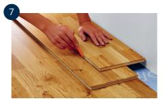
The last row of boards usually needs to be cut lengthwise. Lay the last board with the tongue against the wall, straight across and edge to edge with the penultimate row of boards. Add a piece of scrap board and measure the distance by sliding the board along the wall, while at the same time marking with a pencil where you need to saw the last board. Consider the requisite expansion joint of at least 8-10 mm.
