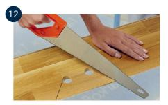
If the long side of the board meets a pipe, drill a hole with a diameter of at least 16 mm larger than the pipe's diameter, so that there is an expansion joint around the pipe. Use a pencil to mark where you want to saw. Saw off the piece to be placed behind the pipes, closest to the wall. Cut at an angle as shown in the picture. If the pipes are located at the short side of the floor, cut the board at a 90° angle straight through the holes.
