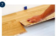
Fold the board down in a continuous motion while applying light pressure on the short end of the previous board. Make sure that the boards are close together when folding down. Continue to install the floor as described previously.
