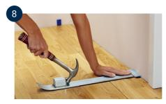
Knock in the sawn-off board using the percussion iron. If the last row of boards has not been cut, the tongue must be cut off so that the expansion joint does not disappear.
