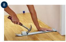
Knock in the sawn-off board using the percussion iron. If the last row of boards has not been cut, the protruding lip must be sawed off so that the expansion joint does not disappear. Also put wedges on the last row of boards. Leave the wedges in place for a couple of hours (e.g. overnight) before removing them.
