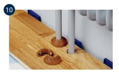
Knock the board into place, glue on the loose piece, place a wedge against the wall and cover with pipe collars.
