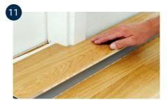
Then install the last board from the side with a percussion iron. Finish by placing wedges in the expansion joint between the floor and the wall, so that the floor has tension until the glue has dried. Now that the floor is installed, mouldings and skirting boards can be fitted; however, do not forget to remove all wedges.
