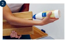
Glue the groove on the short side of the next board using Tarkett Parquet Adhesive D3. Secure the boards using a Tarkett tapping block. Wipe off any excess glue immediately with a damp cloth.
