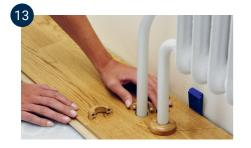
Install the board, glue the loose piece in place, place a wedge against the wall, and cover with pipe collars.
