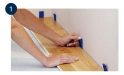
Lay out the first row of boards. Start with the groove side against the wall and work to the right. It is very important that the first row of boards is straight.
