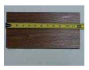
The remaining piece cut from the last plank in the first row may serve as the first plank in the second row provided it is at least 12 inches (304mm) long. Always stagger end joints from row to row a minimum of 12 inches (304mm).
