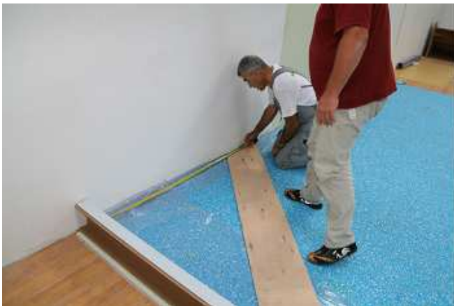
Installation of the first panel of Tarflex
