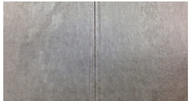
This seam has not been grooved deep enough. The jute backing has not been exposed. The weld rod will likely pull out when trimming or after installation resulting in failure.
