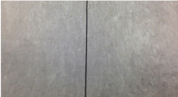
The seam should be cut with a maximum 1/64" gap. Approximately the thickness of a business card.
