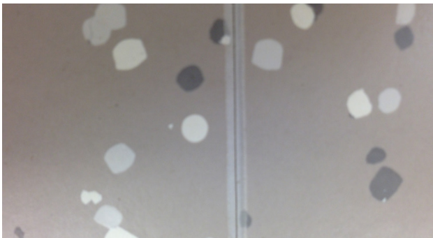
Example of a seam that has not been grooved deep enough. This will result in failure over time.
