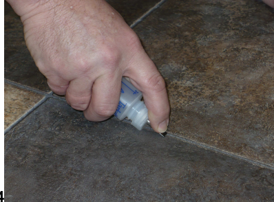
14 Seal seam with recommended Tarkett seam sealer. Protect seam from traffic for minimum of 3 hours.
