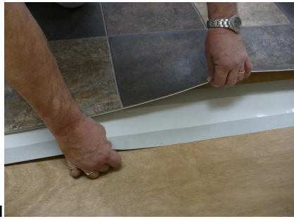
11 When installing over plywood position Tarkett S870 Floating Seam Tape so it is centered under seam cut.
