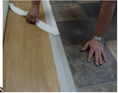
12 Remove release liner from seam tape.
