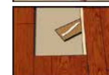
Picture 7: Preparation of layers is done by spreading glue on a thin laminated foil, or on a piece of veneer, first spreading the glue on veneer below the neighbouring boards, and after that spreading glue on a part of veneer which should fix the new board.
