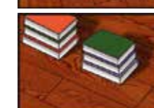
Picture 10: Use weights to press it down for at least three hours, to be sure that the board is well fixed – glued on neighbouring boards.
