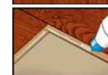
Picture 8: After that spread the glue on a free profile of neighbouring boards and on tongue on board.
