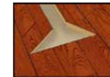
Picture 4: Remove the short ends, and then remove the long sides which are connected with neighbouring boards.
