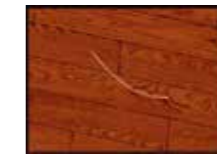
Picture 1: In case of serious damages of your wooden floor (scratches, or damages resulting from impact of heavy or sharp objects), the easiest and the most efficient way to repair it is to change damaged board.
